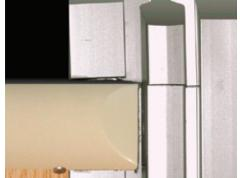
BEST Hospital Tip Caps assist in preventing the hanging of objects on the tip of the hinge. Our hospital tip caps provide a custom fit for each hinge model ensuring the ideal look and functionality. All models are designed to mitigate ligature points whether the door is in the open or closed state.
